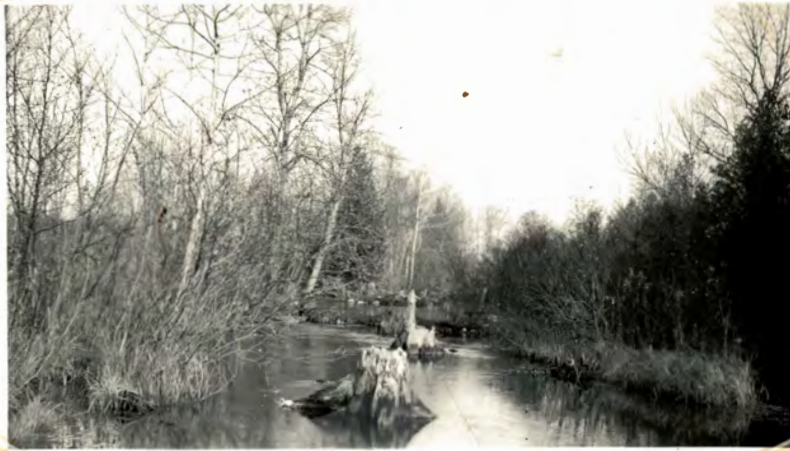
North Branch Au Sable near Boutell's cottage. These wing deflectors should do good work, although the sod should be held on with binding poles. Digging logs at end are of questionable value.
