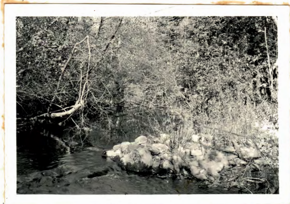
Four year old log and boulder wing deflector in Mackinac County, Black River. This is one of the best possible types of construction if necessary materials are available.
