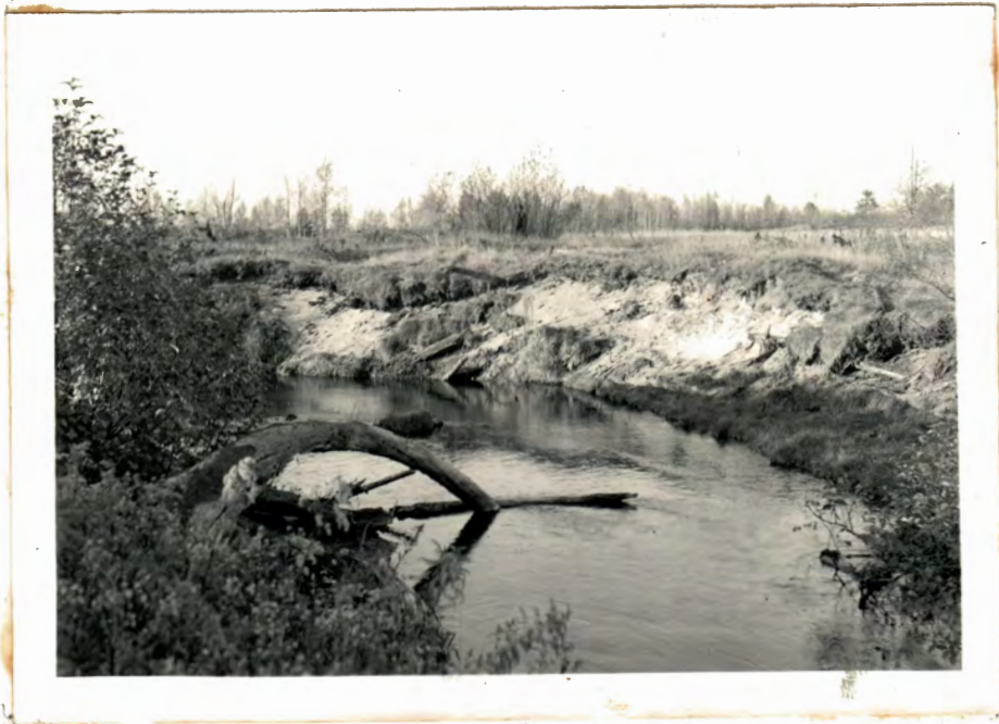
Sod covered bend raft in Carp River near Brevort. Unless sod is wired down it is certain to be damaged and stripped away by ice and high water.
