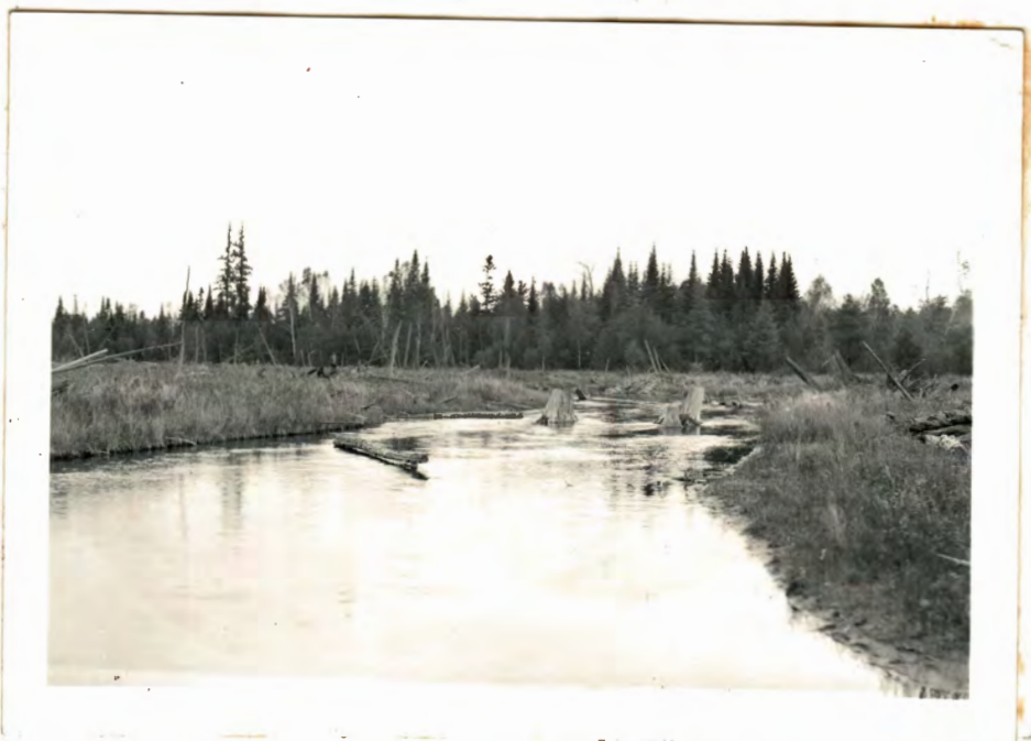
Log and stump barriers in Manistee River west of Gaylord. In the main, these structures are in harmony with their surroundings, and seem to be performing as expected. Isolated digging logs, as seen in the foreground, are of questionable value.
