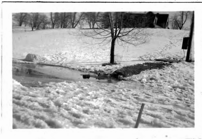
Figure 17. Open hole produced by pumped water.
