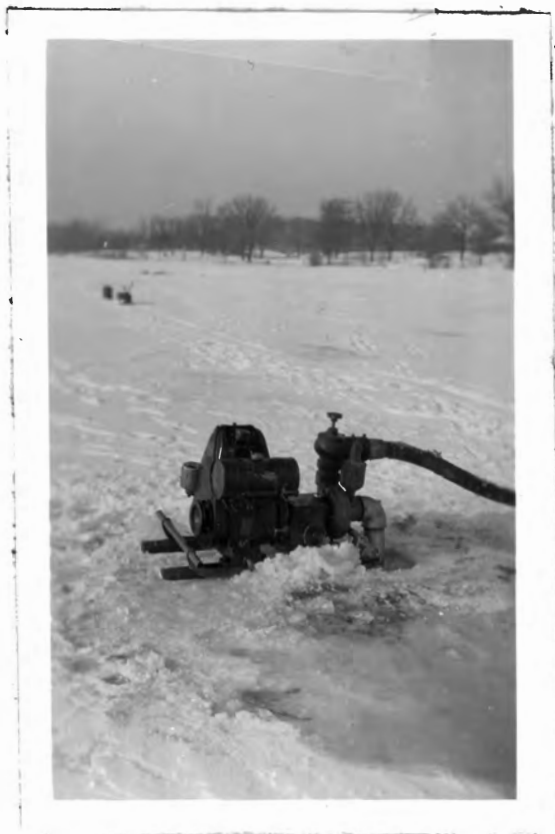
Figure 5. Pump and motor.
