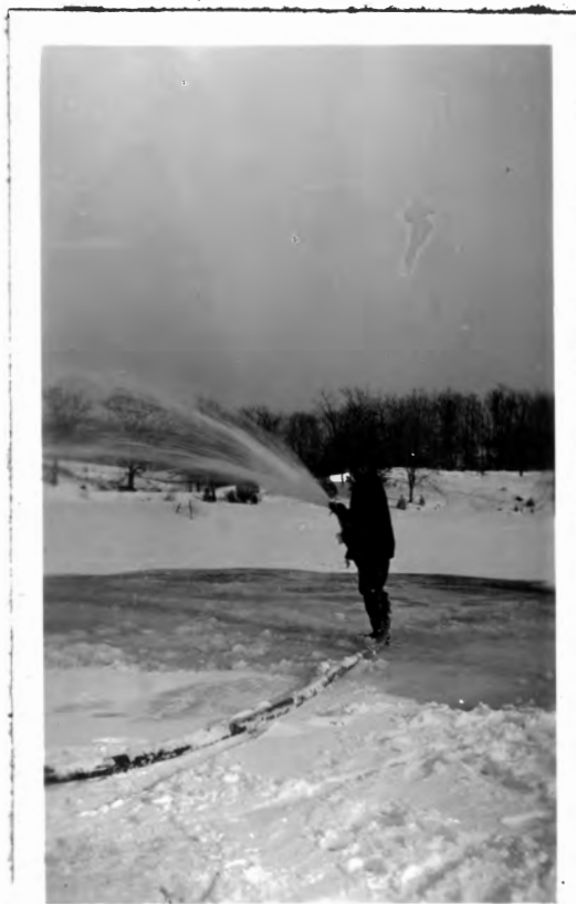
Figure 6. Pump discharge by spray.
