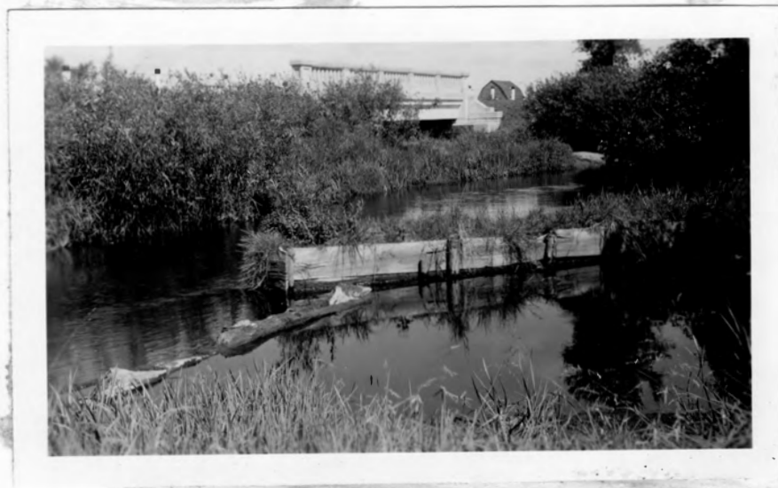
Fig. 25. Upstream view of area behind old deflector, Clam River. Excellent silt bed containing hundreds of nymphs, which shows indications of becoming filled in and grown over to form solid ground.
