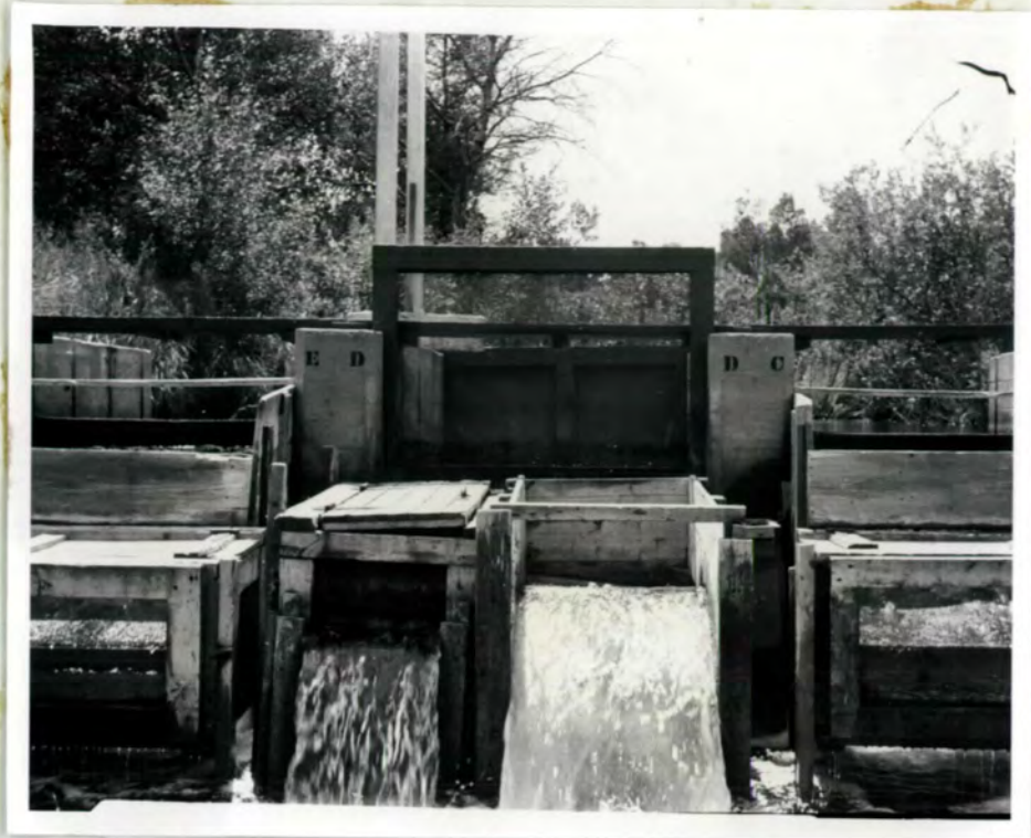
FIGURE 8.--Section Z bulkhead. A close-up of the downstream side of the down-trap holding box (left center) and the falls created by the new up-trap (right center).
