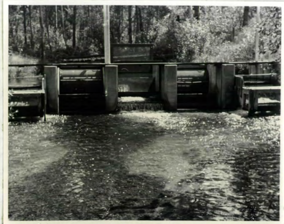
FIGURE 3.--Section D bulkhead looking upstream. The center slot contains the V-shaped up-trap, here in operation.
