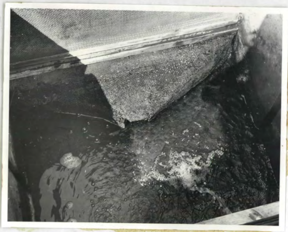
FIGURE 3.--Section D bulkhead looking upstream. The center slot contains the V-shaped up-trap, here in operation.
