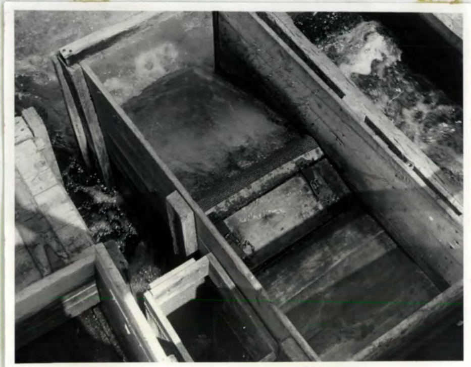
FIGURE 9.--Section Z bulkhead. Looking down on the new up-trap showing the inclined boards which direct the fish into the small holding box at the lower center of the picture. The down-trap holding box is at the upper right, and a portion of a Wolf trap is at lower left.
