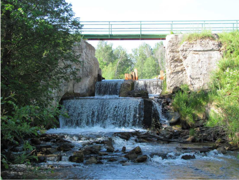
Photo 1. Manton Millpond Dam prior to removal.
