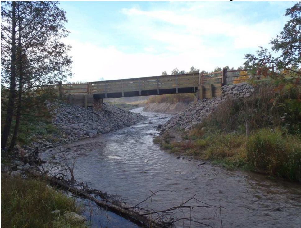
Photo 2. Manton Creek after the removal of Manton Millpond Dam.
