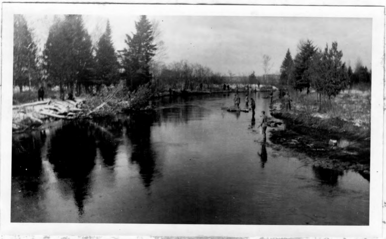
Plate 2. Downstream view from U.S. 2 bridge; 9:00 a.m., April 15, 1951.
