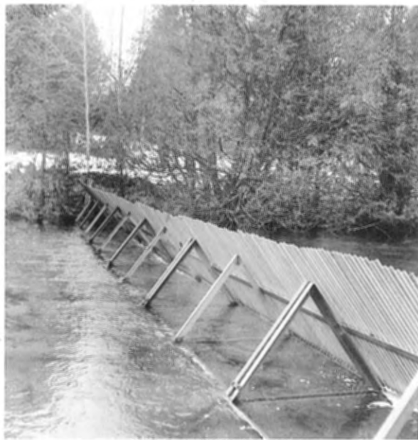
Figure 2.--The fish barrier located above Experimental Section I, showing the downstream side.
