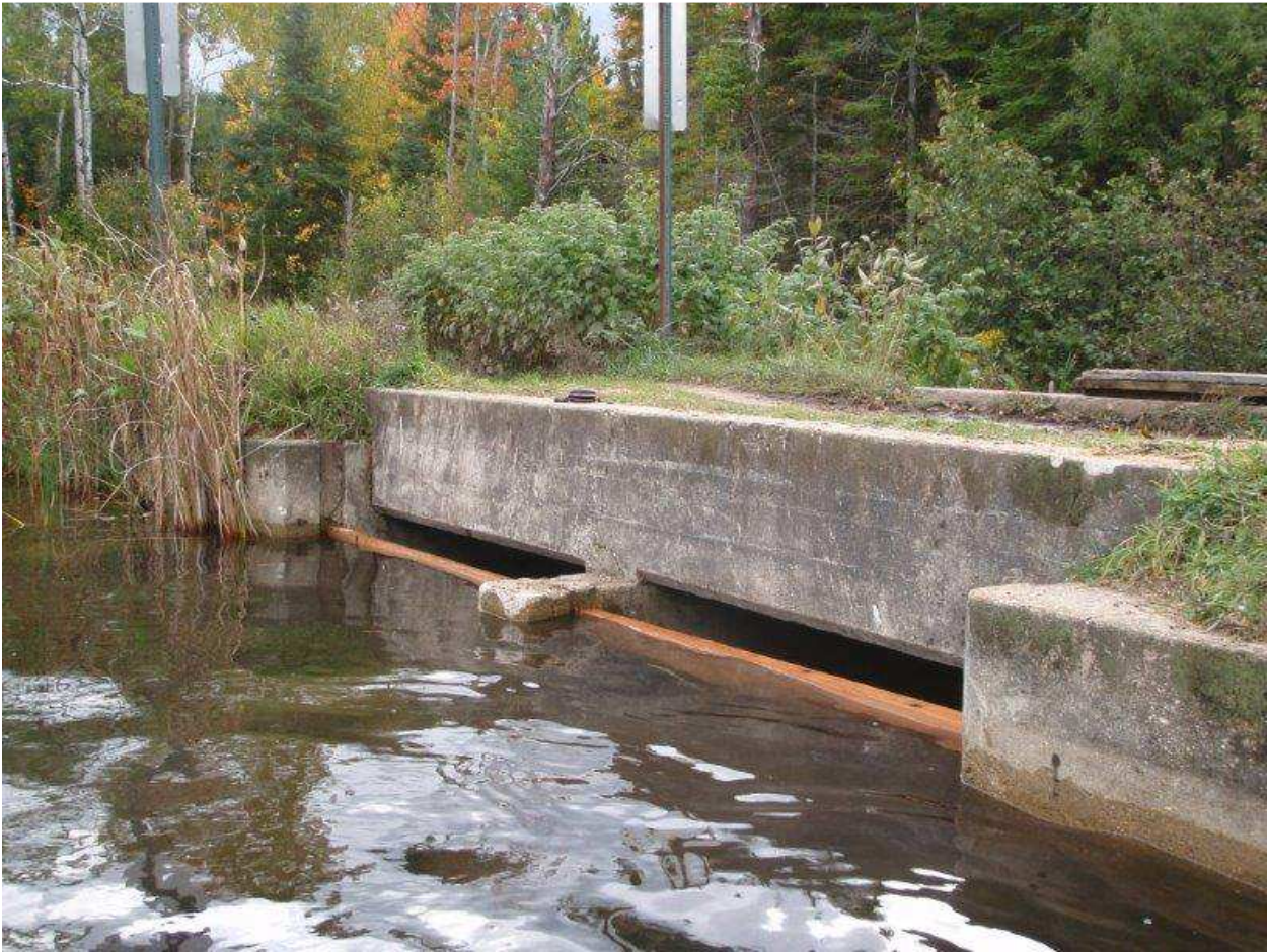
Photo 2. Water Control Structure/spillway 2014 following board maintenance.
